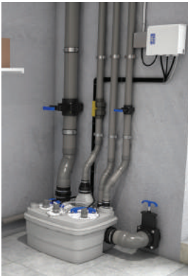
Sanicubic 2 Pro pumping station installed in the basement
