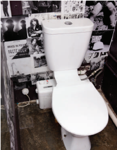
Sanibest Pro installed in basement toilets
