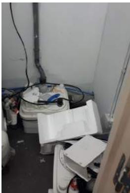
Sanicubic 1 installed
