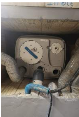
Sanicubic 1 VX installed in the garage
