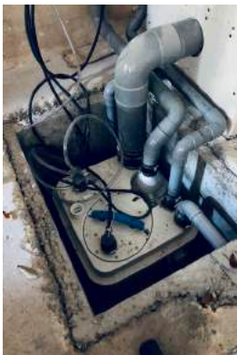
Sanicubic 1 WP installed in the basement
