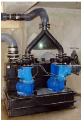
Sanicubic 2 SC installed in building cellars
