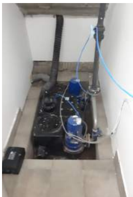
Sanicubic 2 GR pumping station installed
