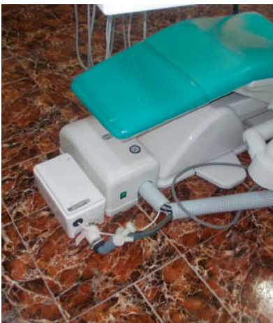
Sanidouche+ pumps installed to drain wastewater from sinks
