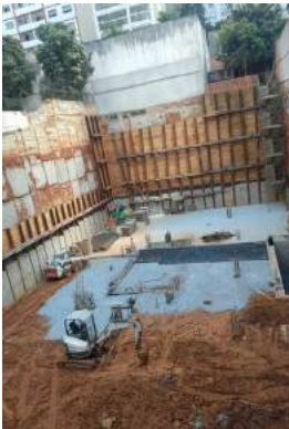
Overview of the site with the installation of the Sanifos 2100
