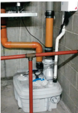
Sanicubic 2 VX installed in the equipment room
