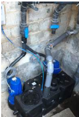
Sanicubic 2 GR installed in place of the old station
