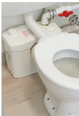
Sanibroyeur Pro Up installed to evacuate waste water from toilets into the main drain
